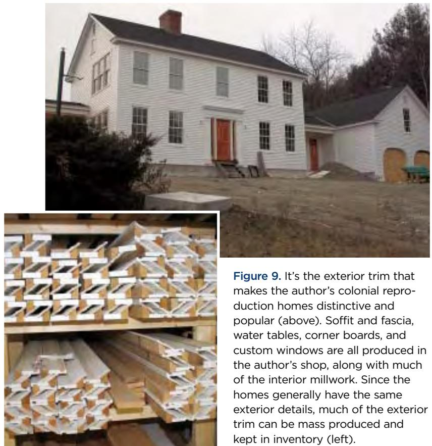
**Figure 9.** It's the exterior trim that makes the author's colonial reproduction homes distinctive and popular (above). Soffit and fascia, water tables, corner boards, and custom windows are all produced in the author's shop, along with much of the interior millwork. Since the homes generally have the same exterior details, much of the exterior trim can be mass produced and kept in inventory (left).
